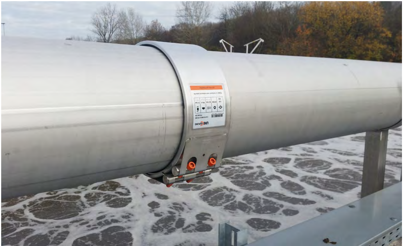
PEWOFLEX 138-F6A4E318-328 PN 10 (Pipe diameter Ø 323 mm, compressed air , EPDM)
